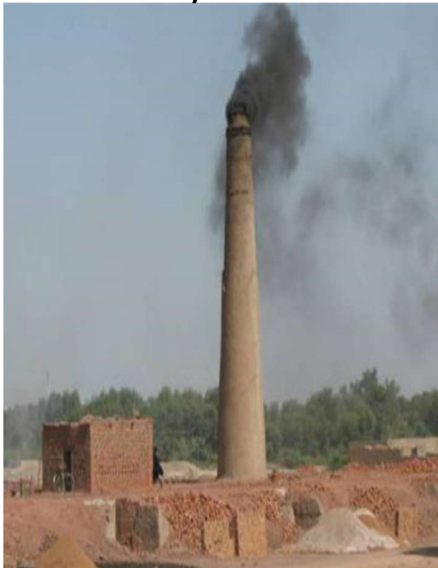
Traditional Brick Kiln System
