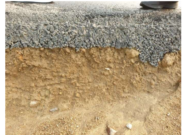
After 6 months Road Layer
